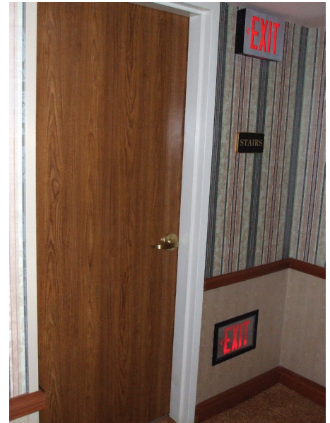
Traditional and low-level exit signs at an interior exit stairway
