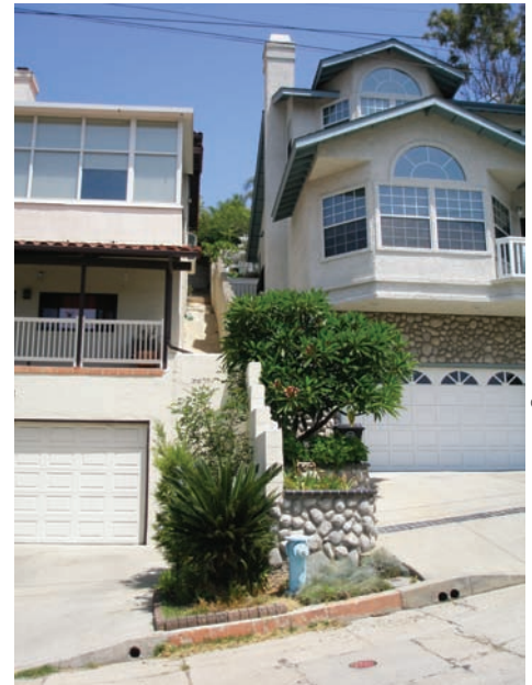
Exterior walls adjacent to lot line.
