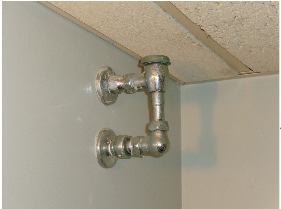
Backflow prevention device (mop sink faucet vacuum breaker—not field testable)
