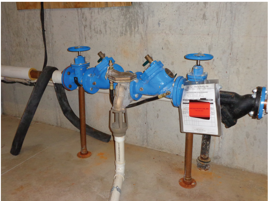
Backflow prevention assembly (field testable)
