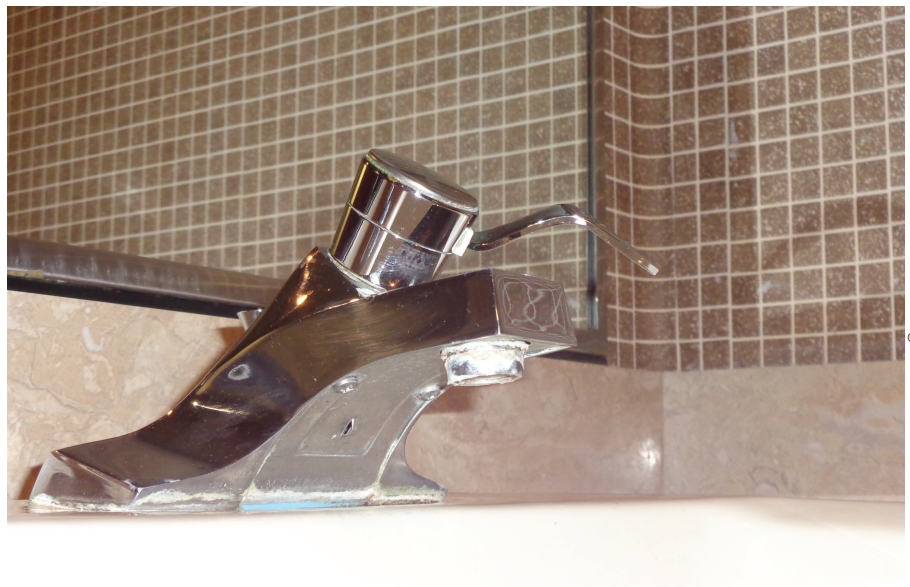
Other means or methods to prevent backflow (air gap—visually inspected)
